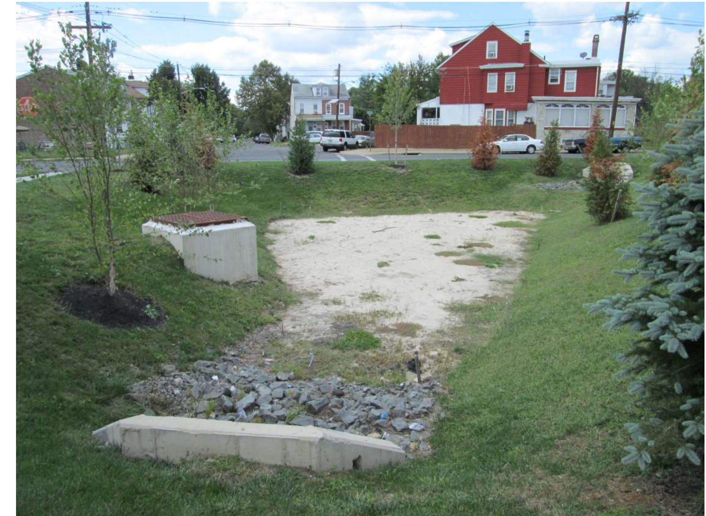
Overview of basin
