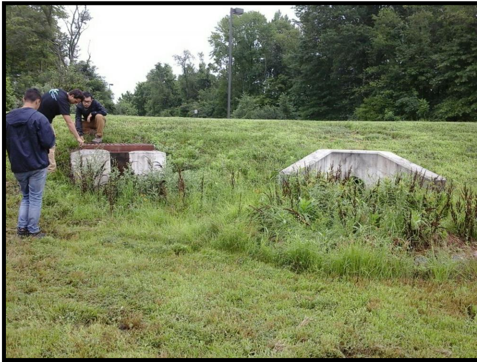
Student interns measure outlet structure at a Route 524 basin
