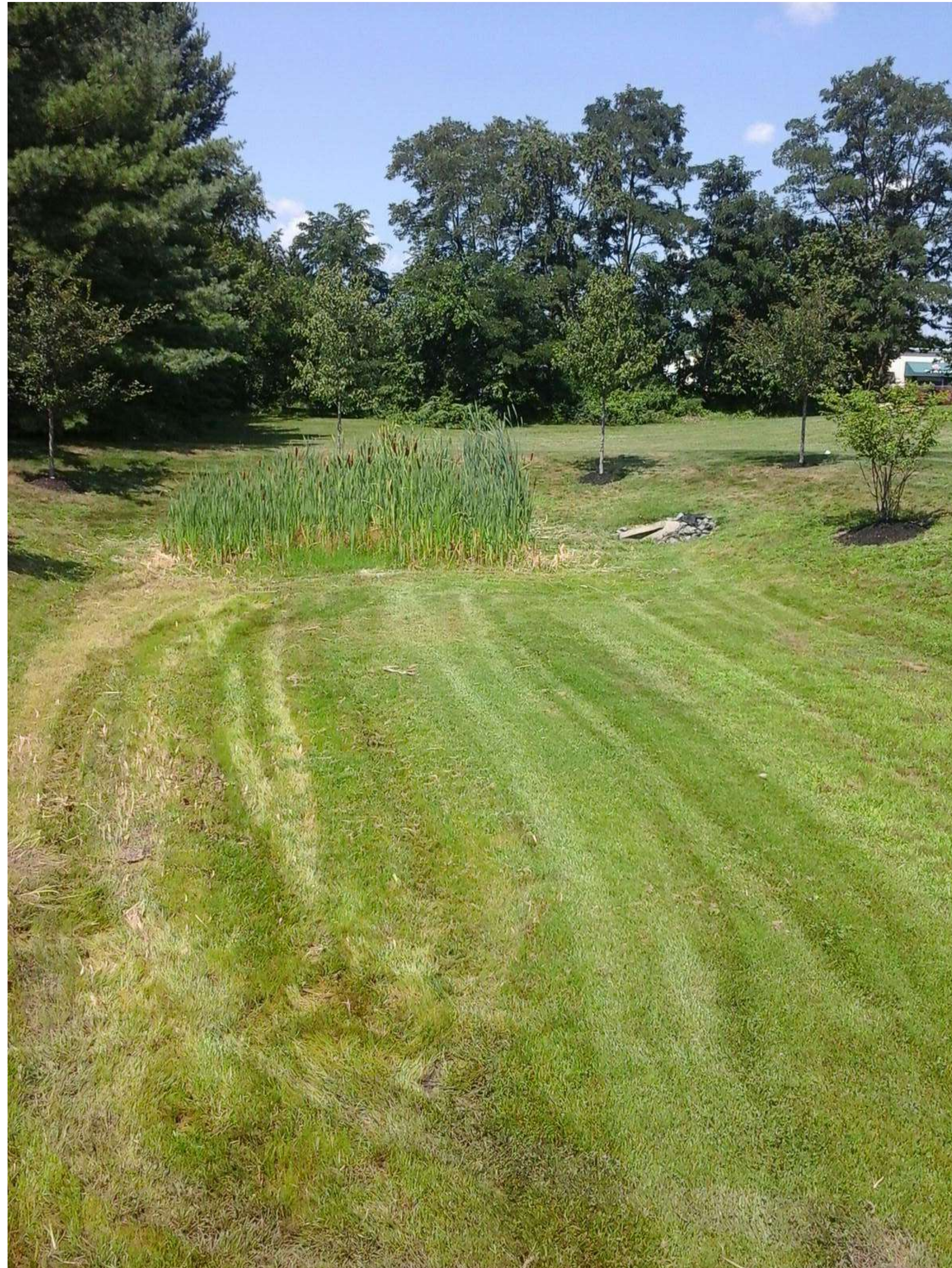
Overview of basin
