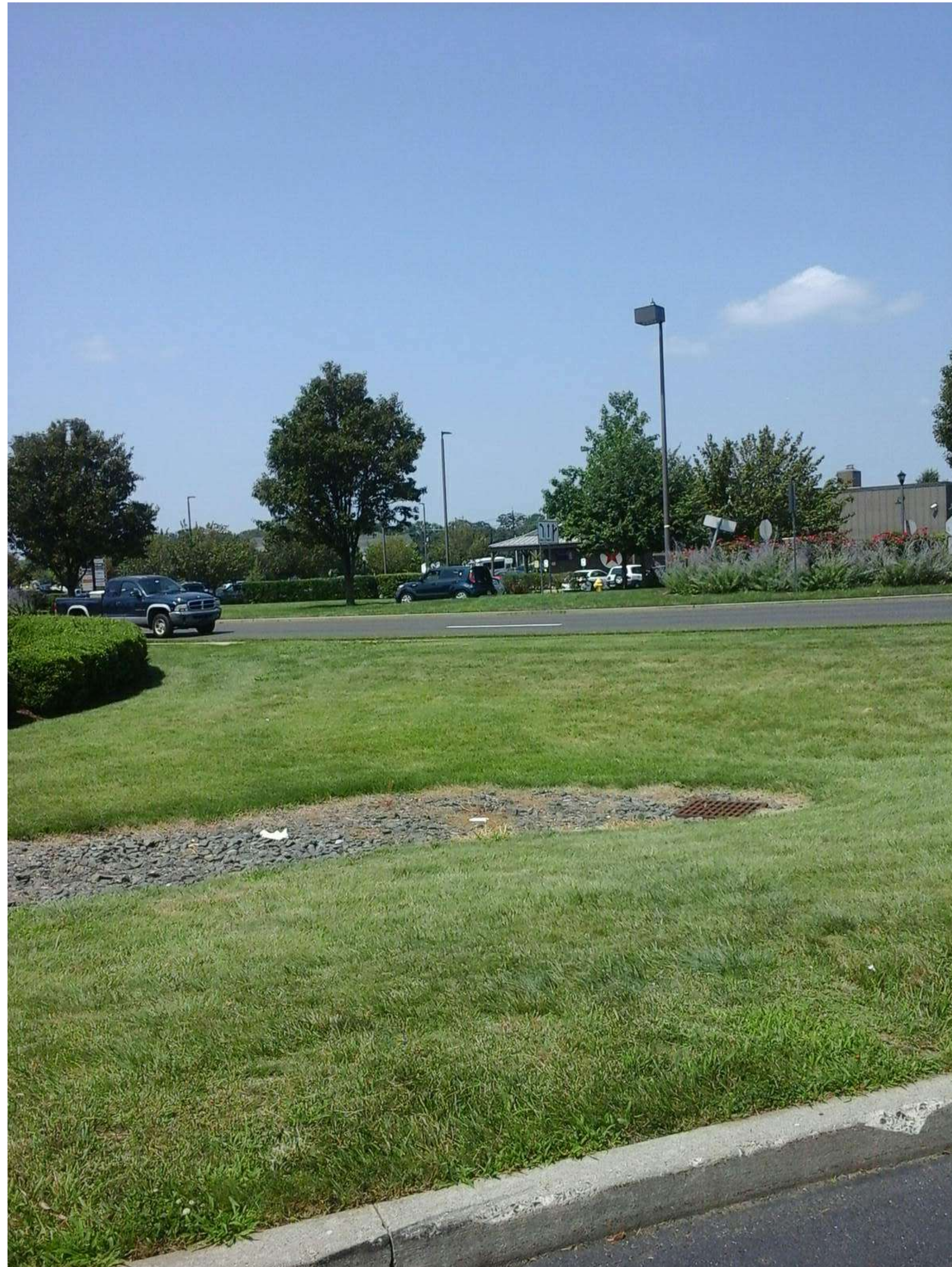
Overview of basin
