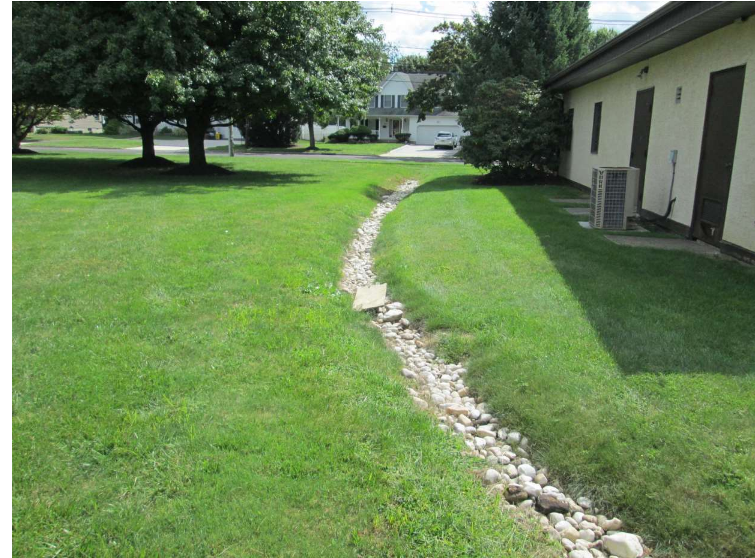
Overview of channel
