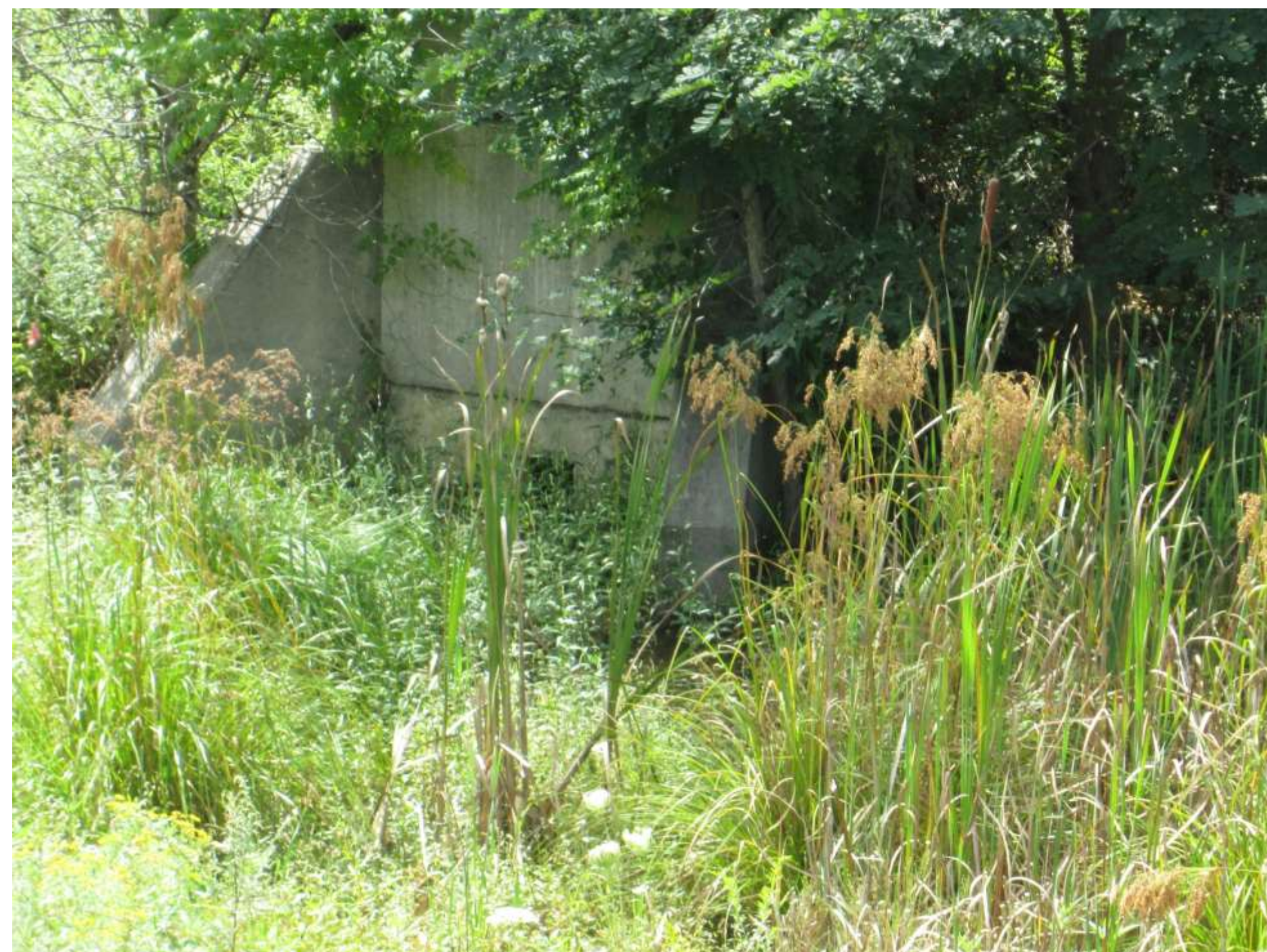
Southern basin overview and outlet structure
