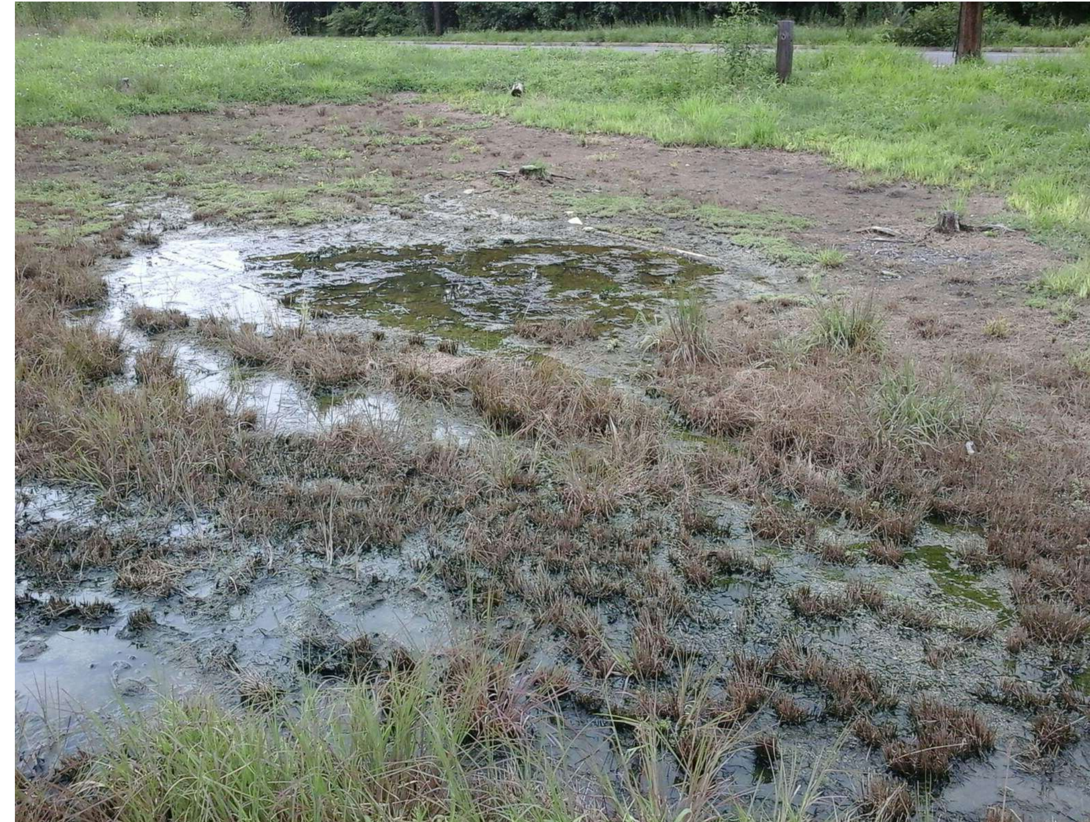
Intlet pipe from road
