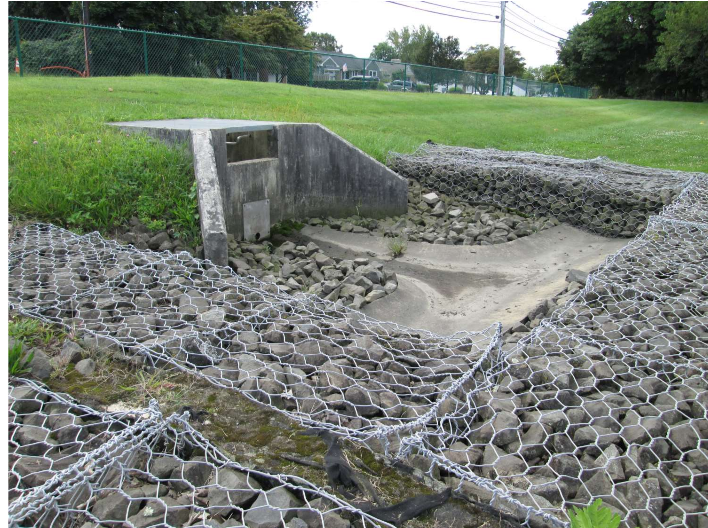
Outlet with gabion baskets
