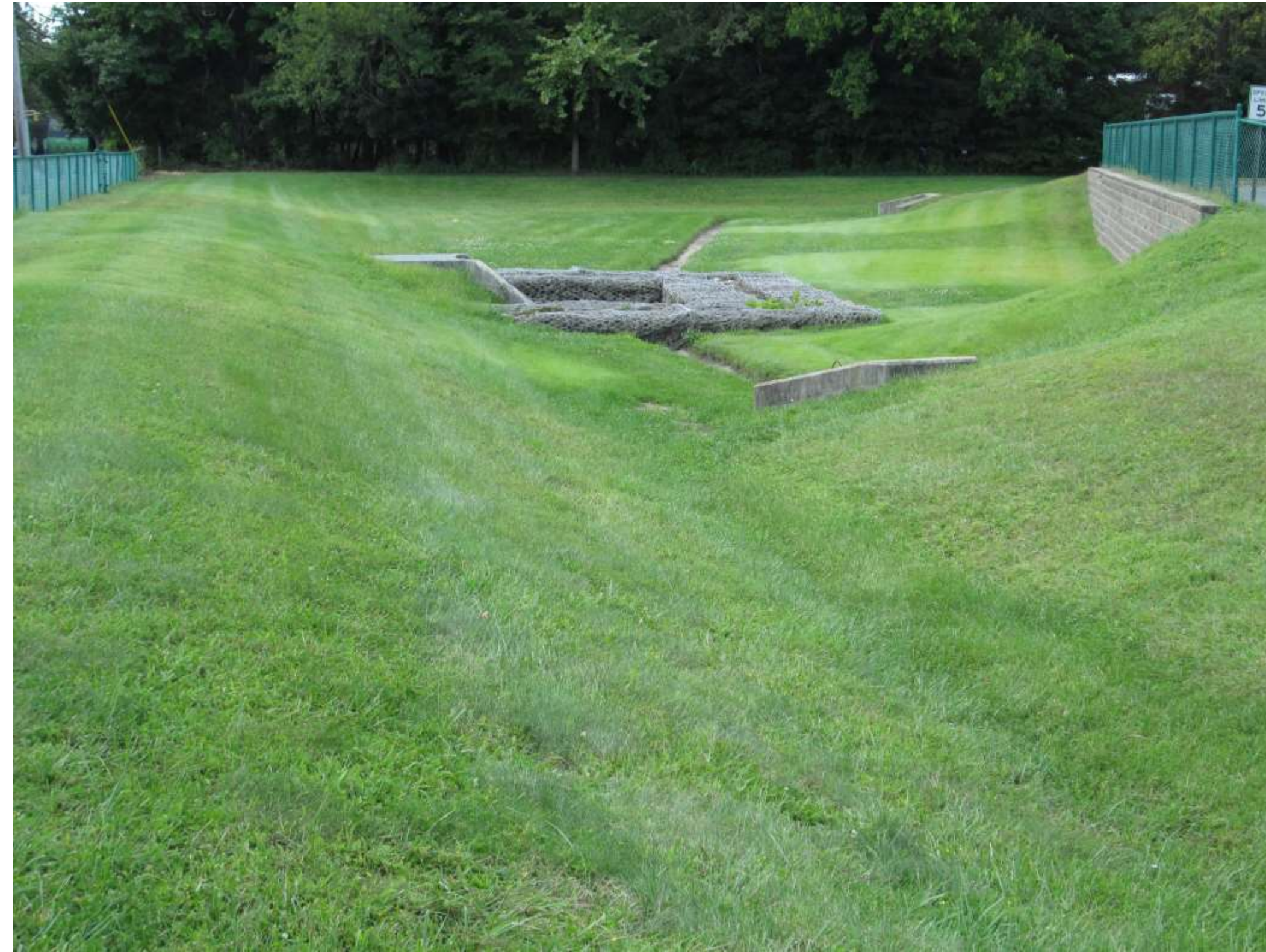
Overview of basin
