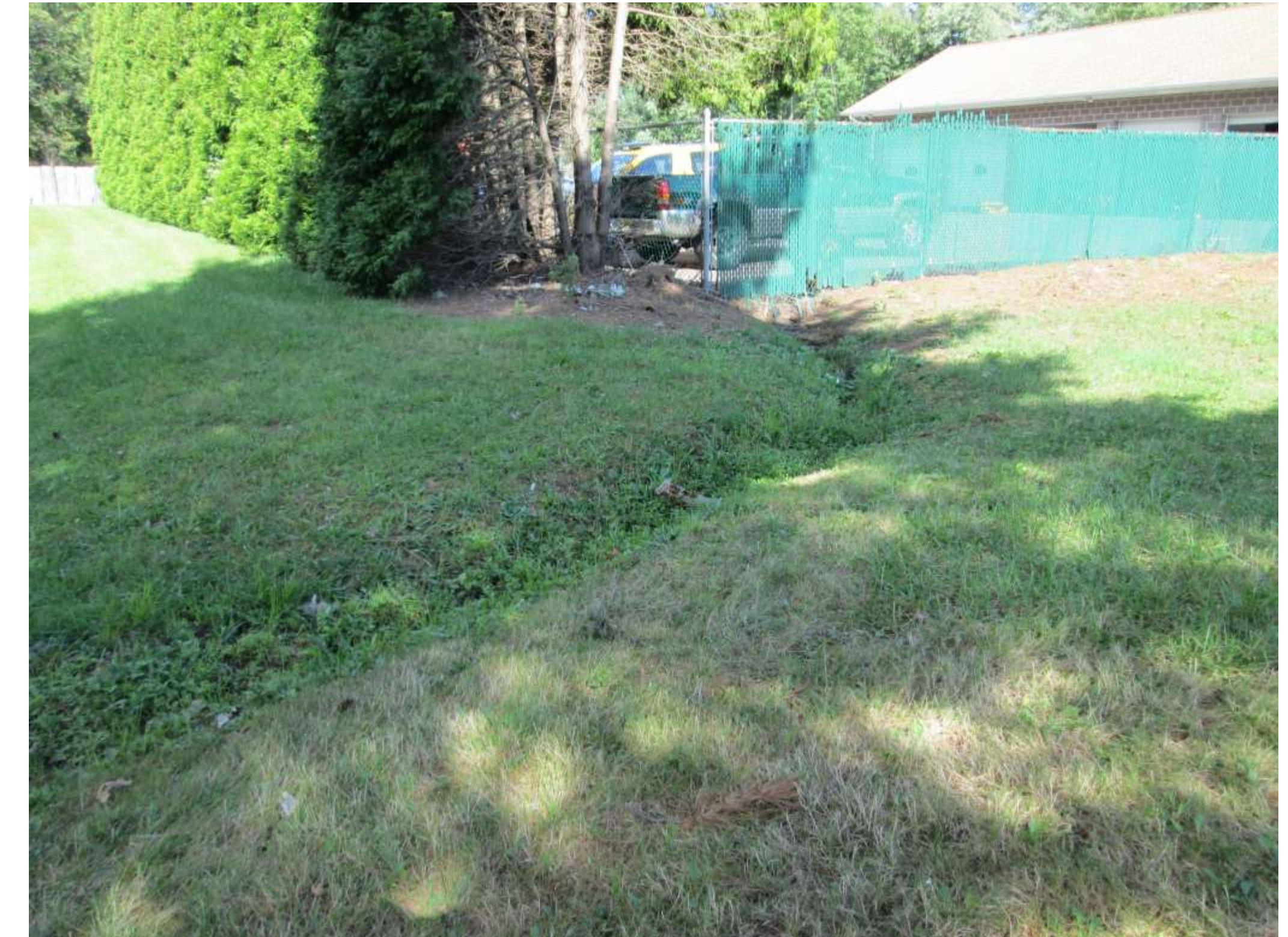
Inlet from parking lot
