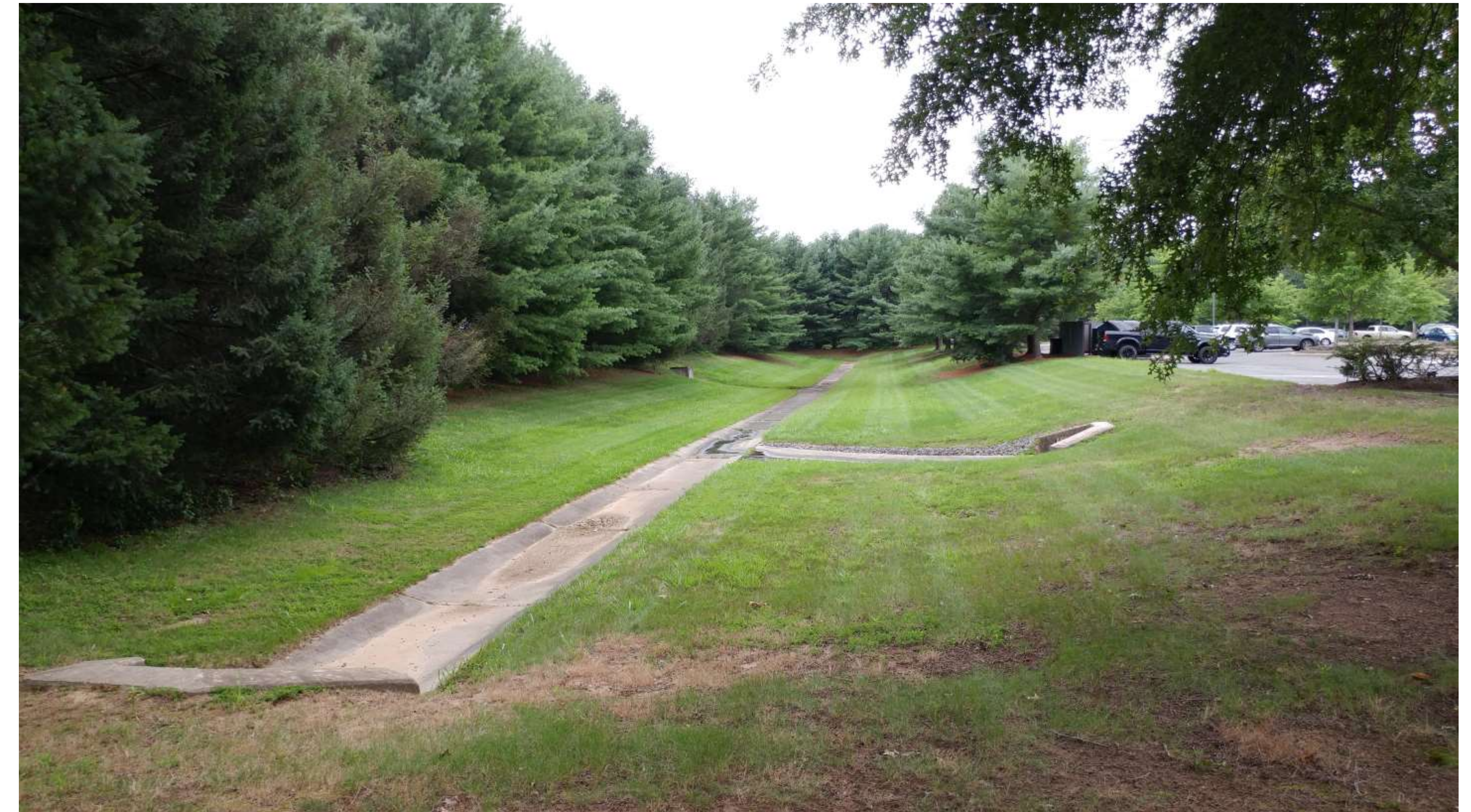
Overview of basin
