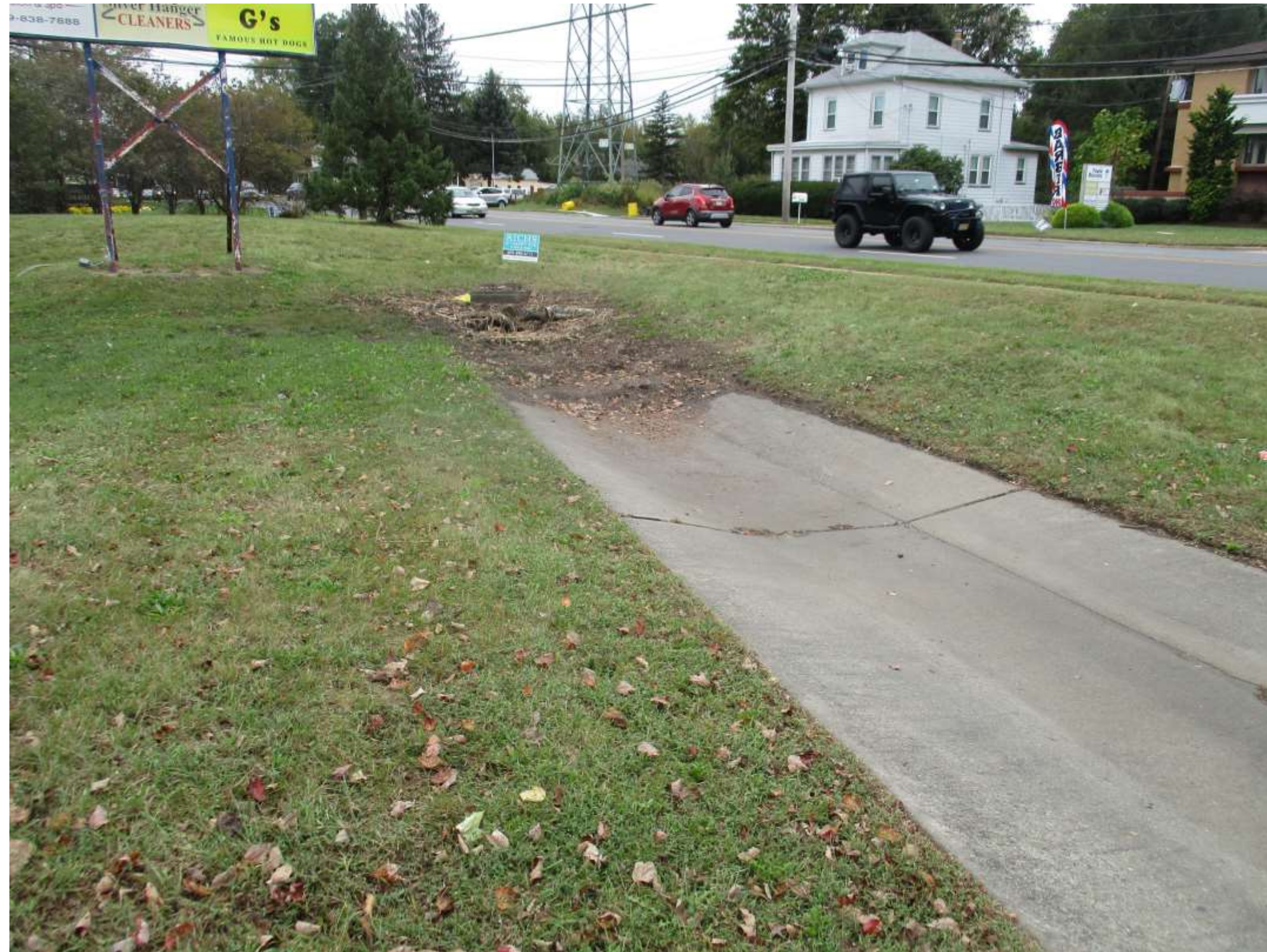
Sediment in low flow channel
