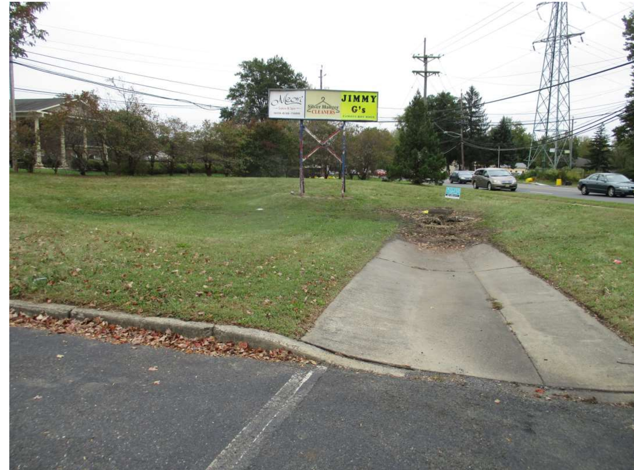
Overview of basin
