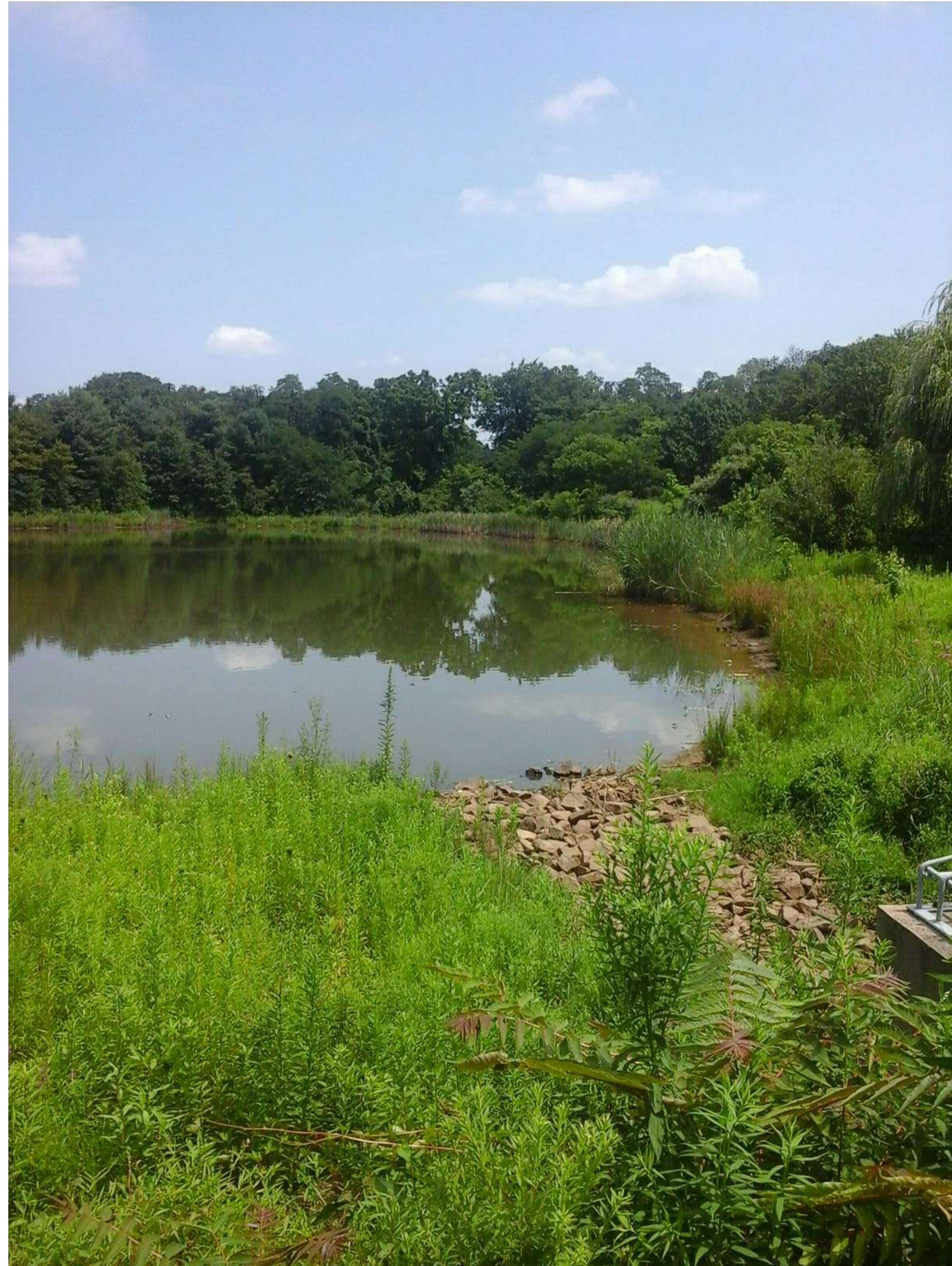
Overview of basin
