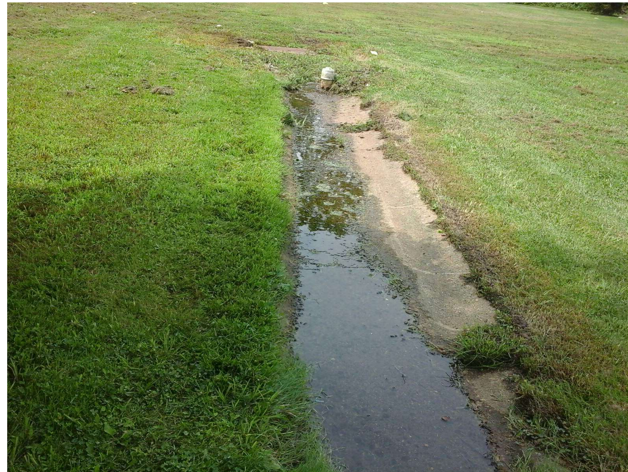
Low flow channel leading to catch basin
