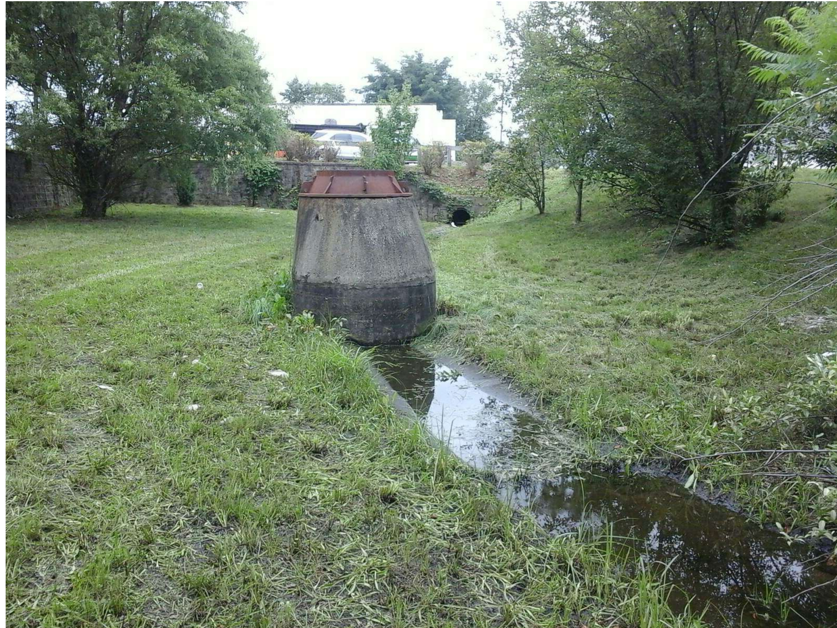
Overview of basin
