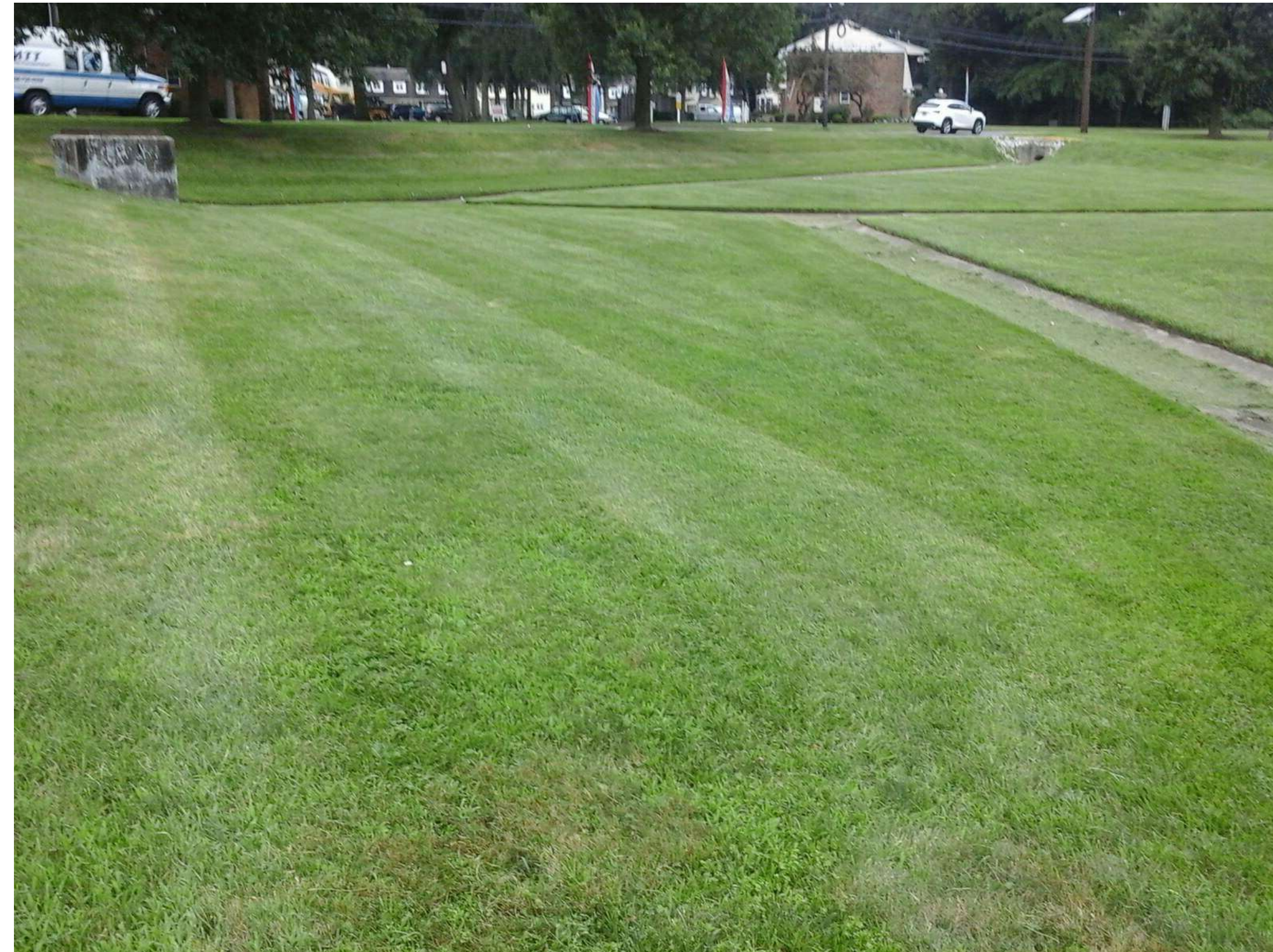
Overview of Basin
