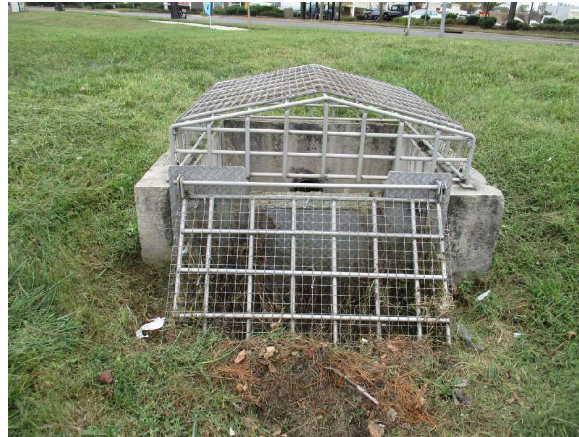
Outlet of 371 (northern basin)
