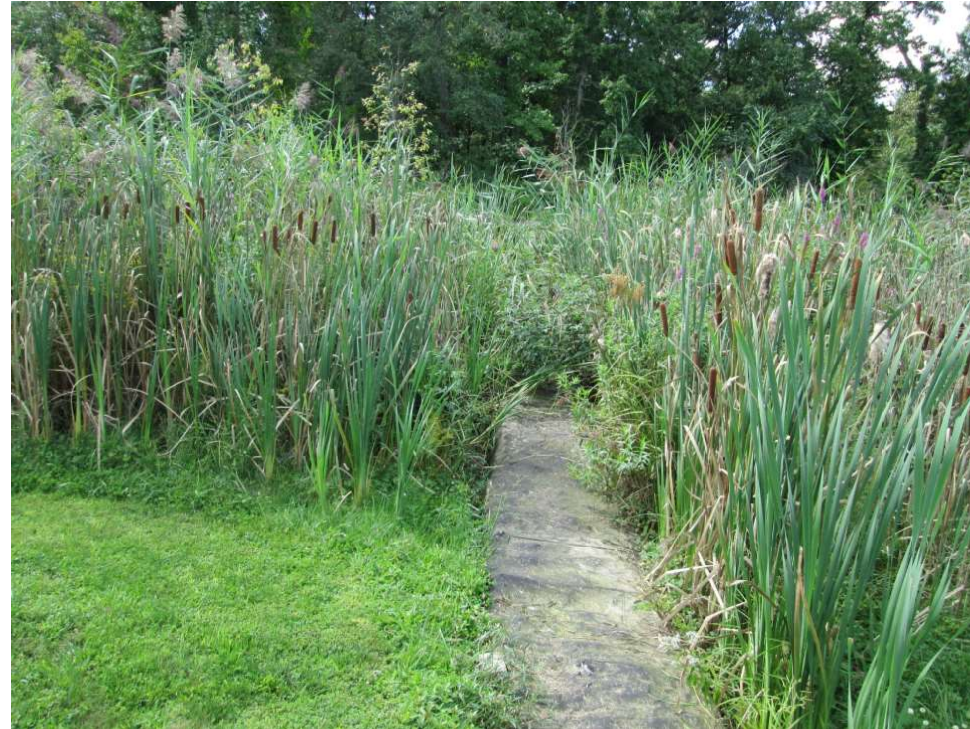
Weir between retention basins
