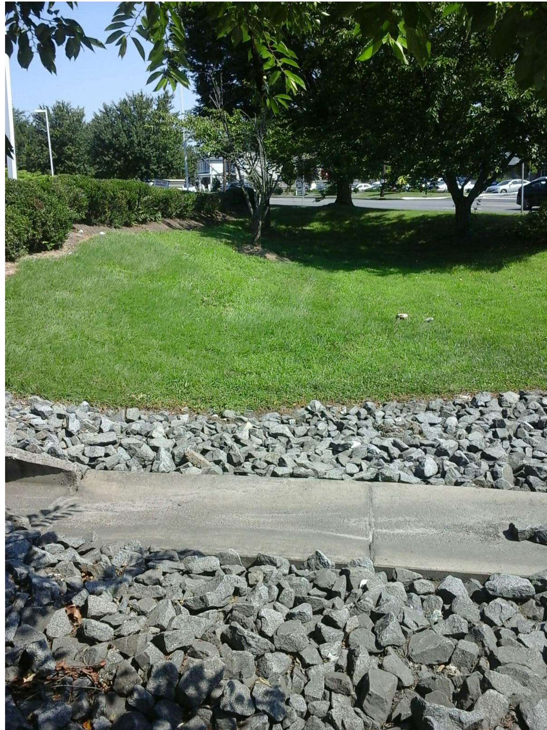
Inlet and low flow channel
