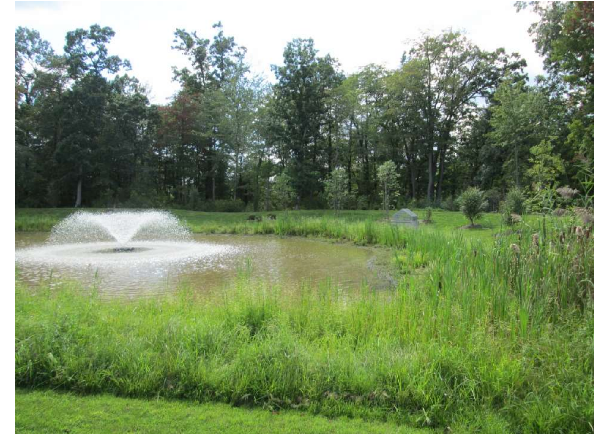
Overview of retention pond
