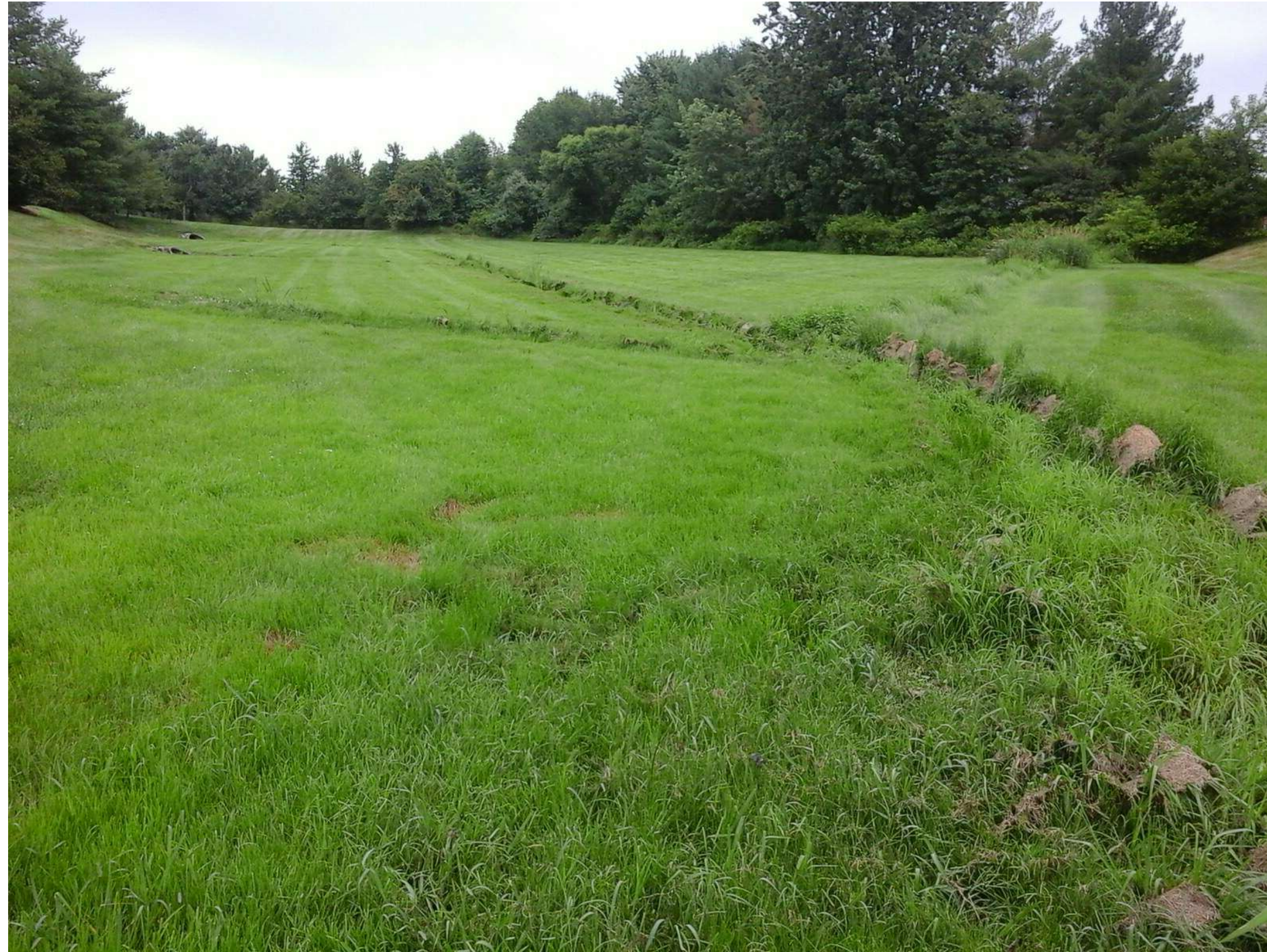
Overview of basin
