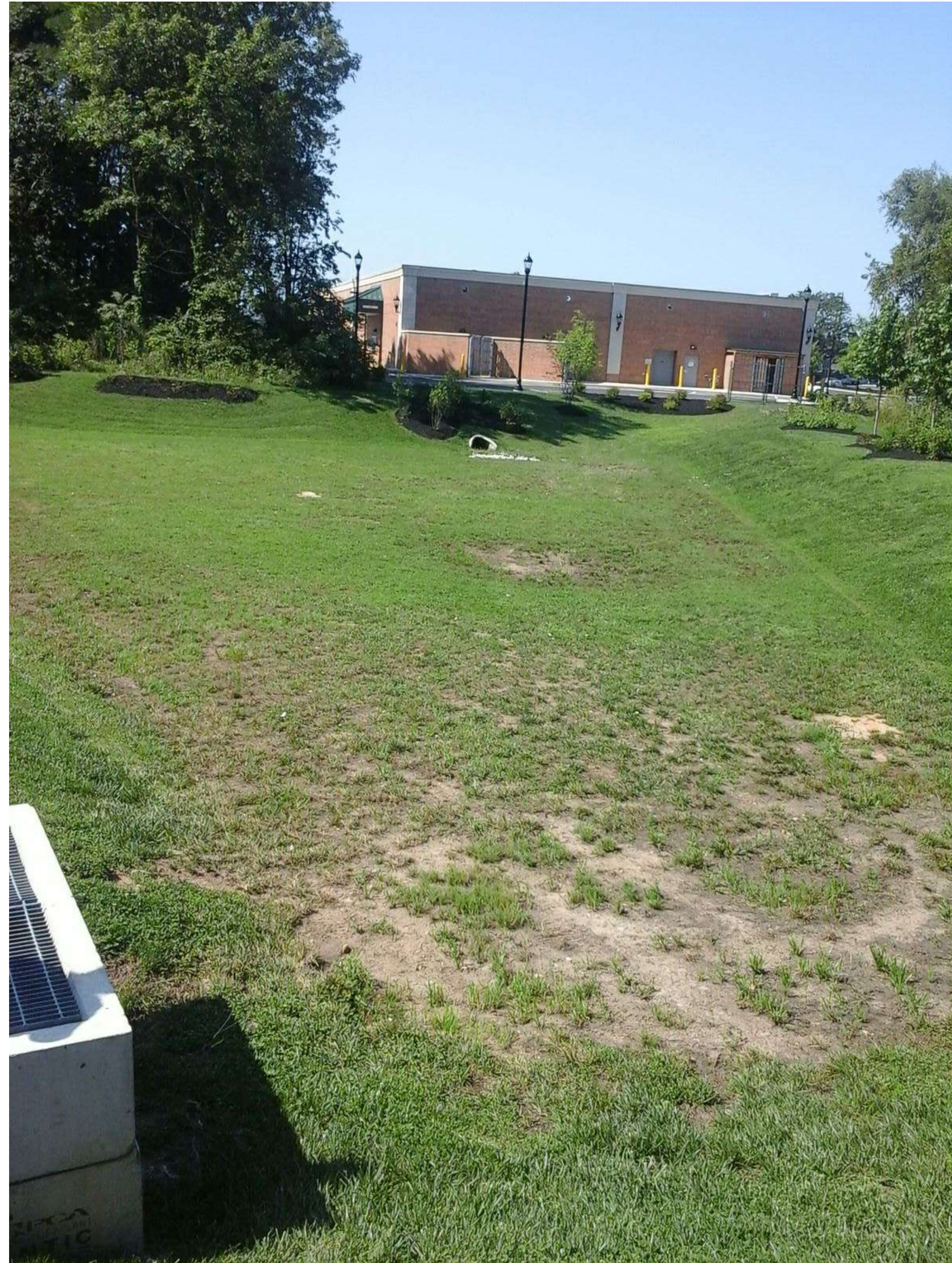
Overview of basin
