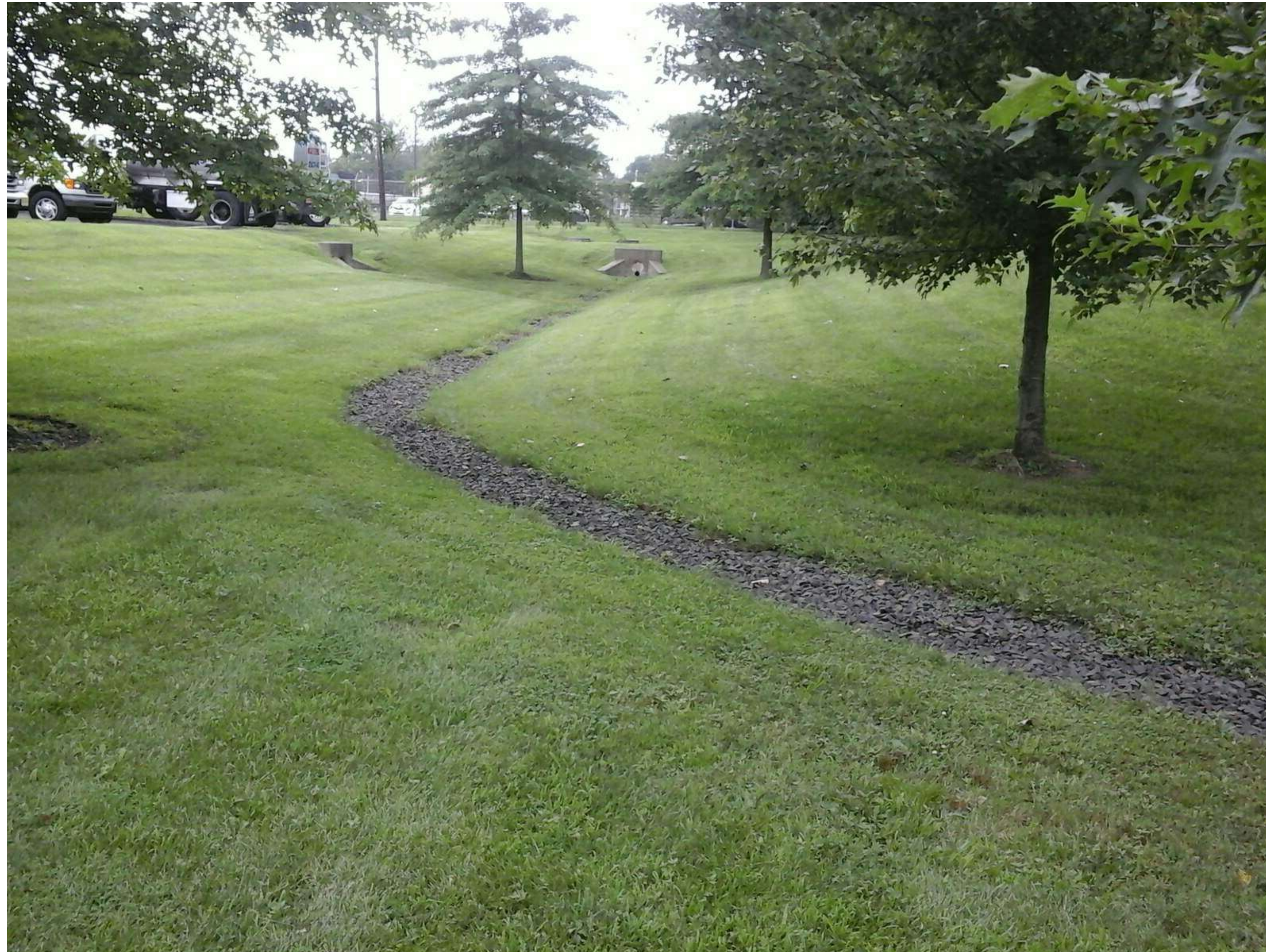
Overview of basin
