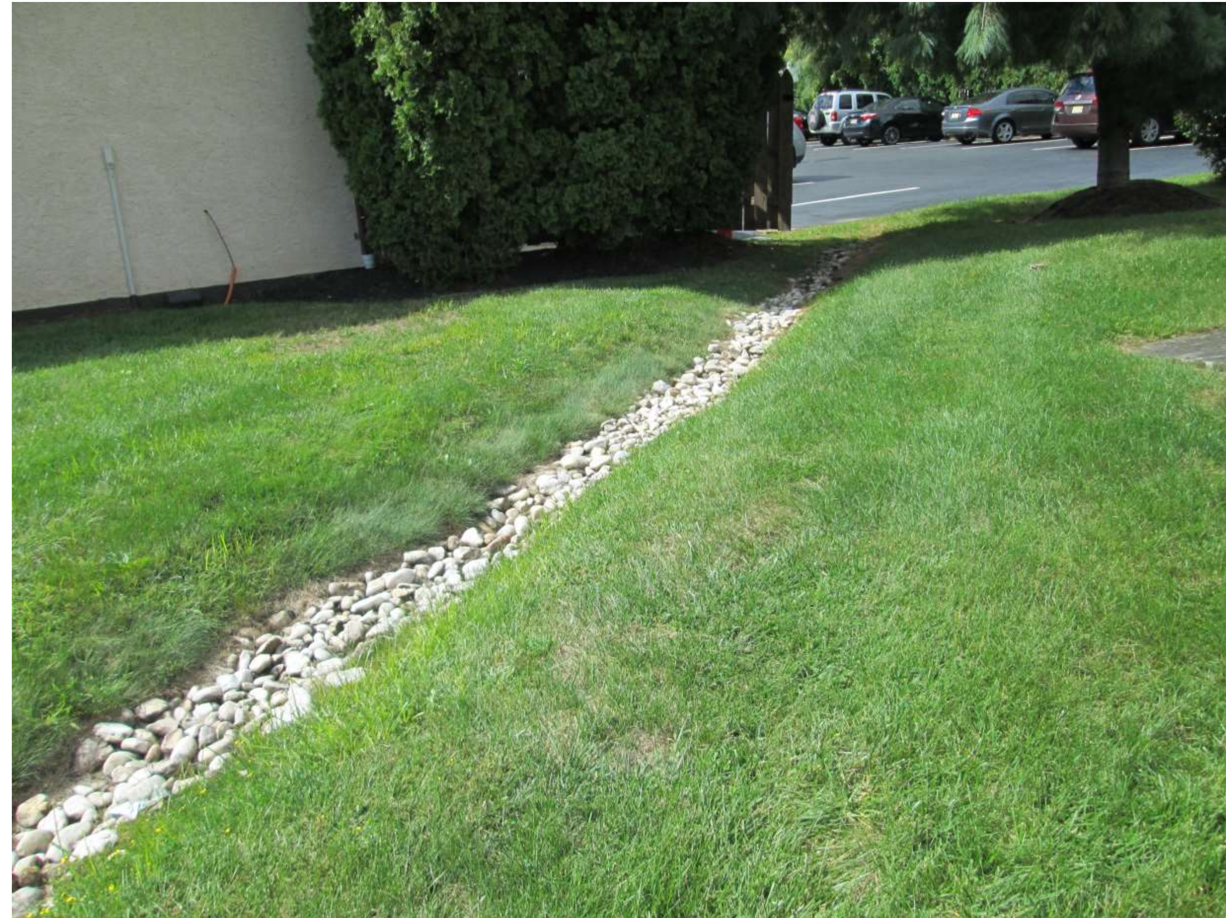
Stone lined infiltration channel
