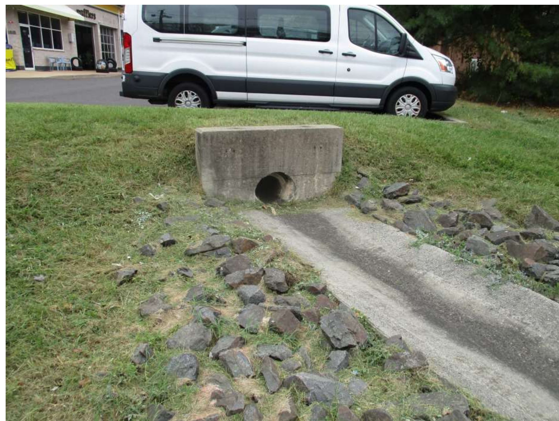
Inlet and low flow channel
