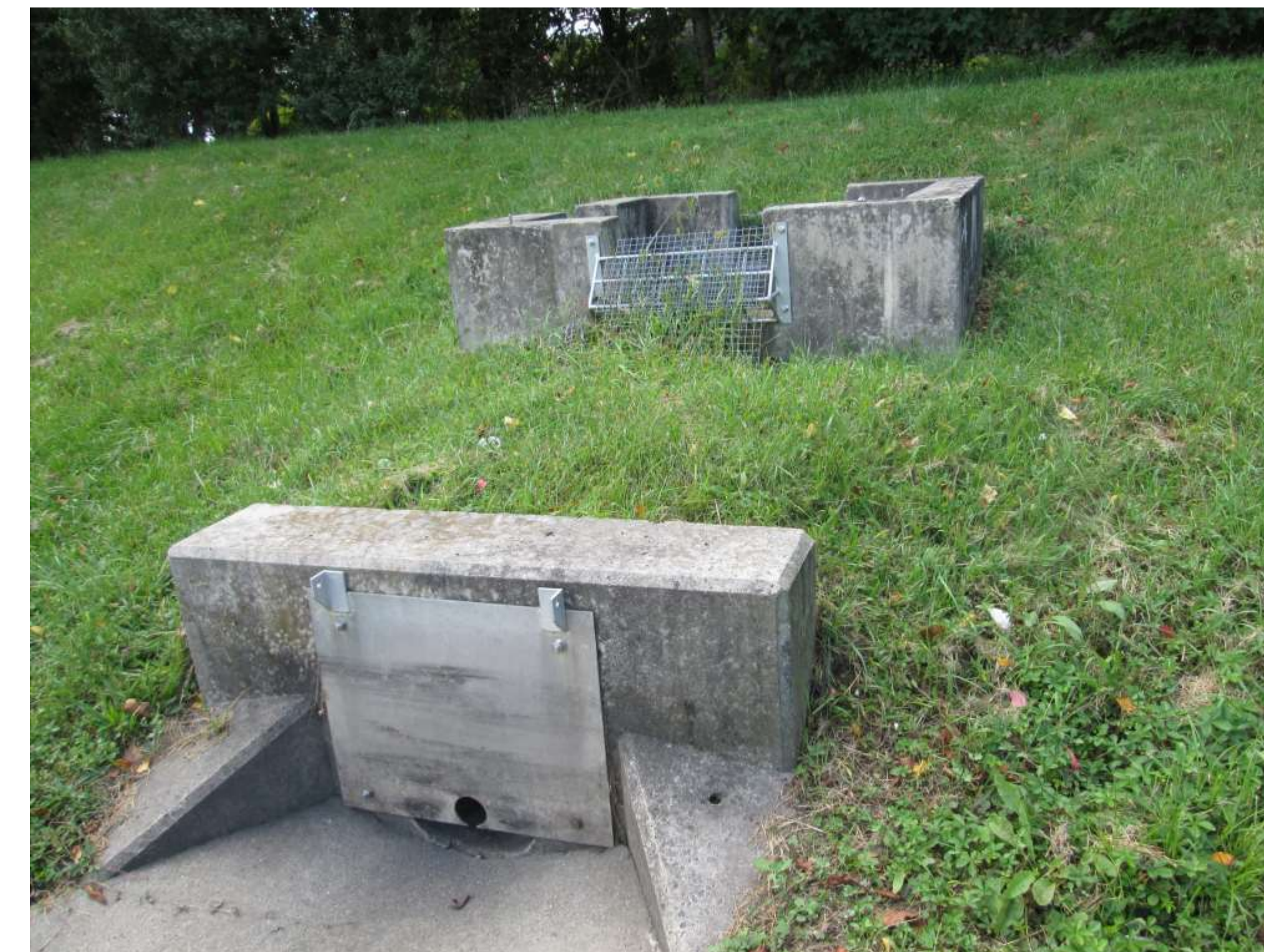
Front view of outlet
