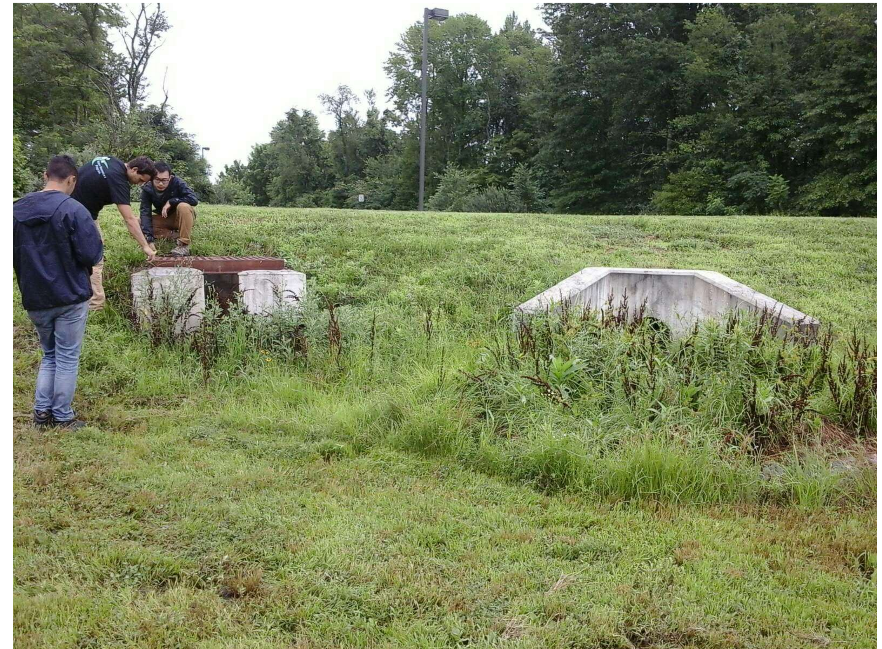
Inspecting outlet structure
