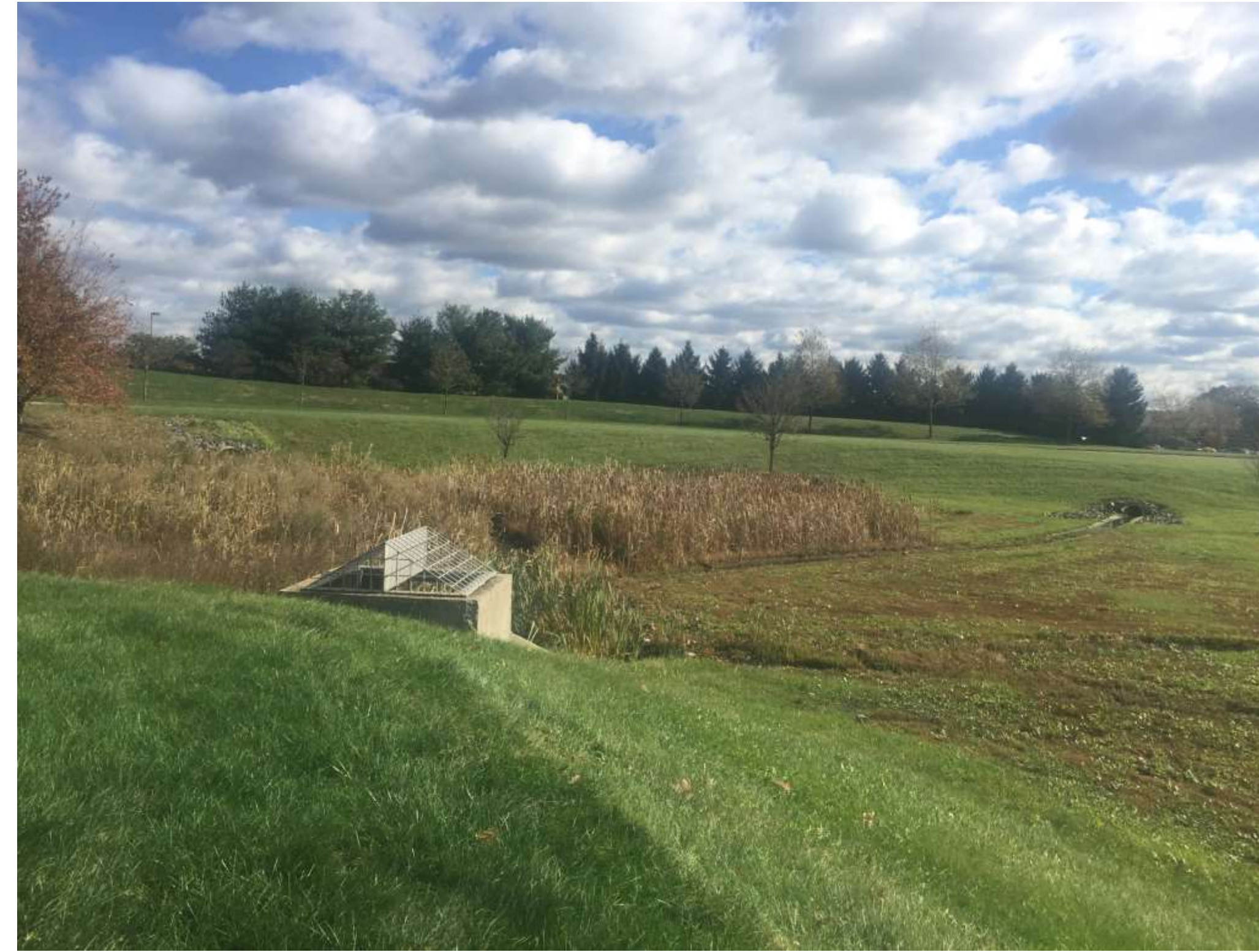
Overview of basin
