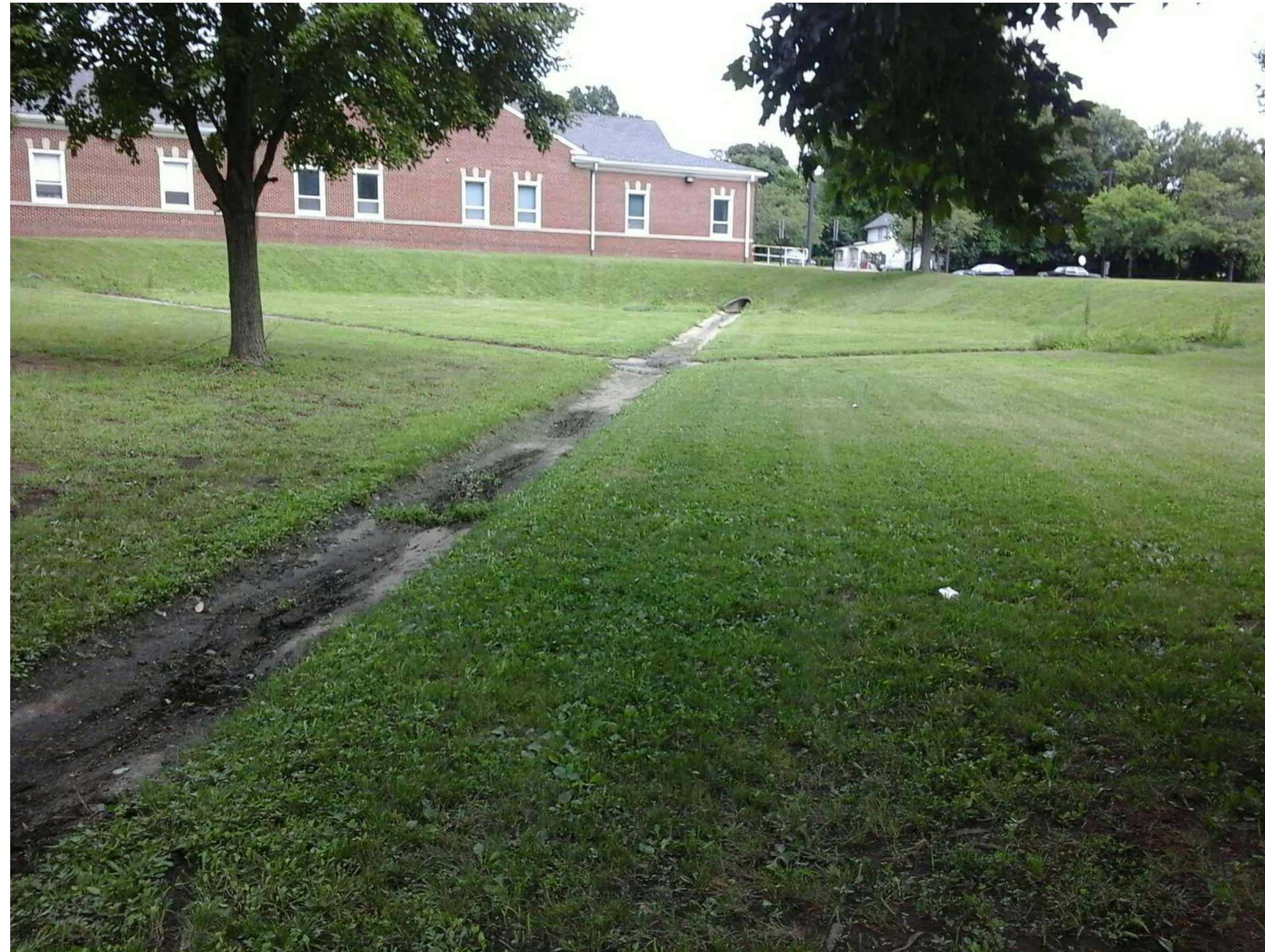
Overview of Basin
